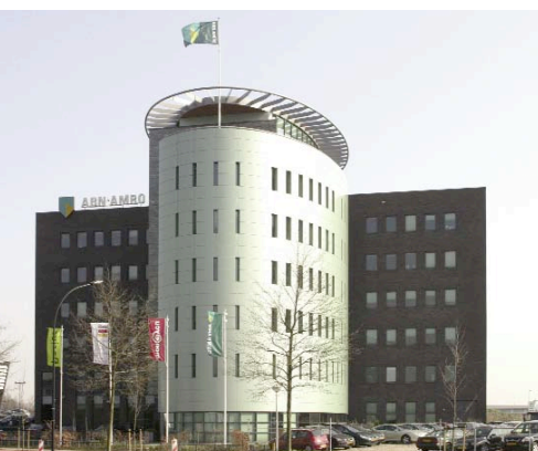
ABN AMRO BUILDING
